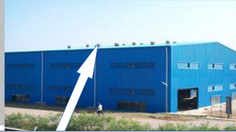
Wind Operated Ventilators
